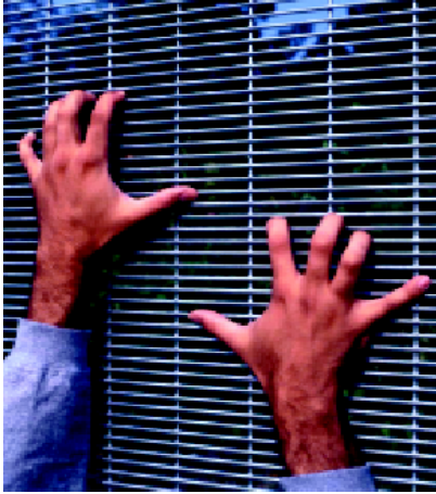
FIGURE 4-9 Fencing with Openings Too Narrow for Adversary to Get a Handhold or Toehold
