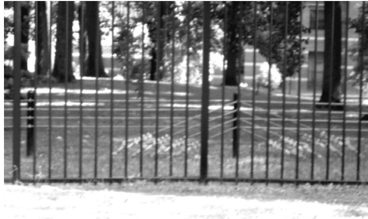
FIGURE 4-5 Perimeter Fence with Aircraft Cable Anchored to Concrete
